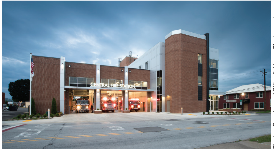
The Russellville Fire Station is a modern interpretation of the existing buildings in the area.
